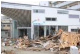
The Kaimashi center after the earthquake
